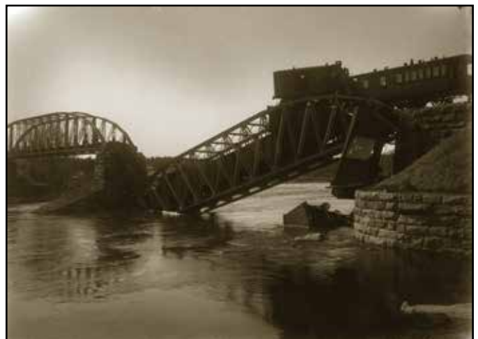
Sabotaged railway bridge
