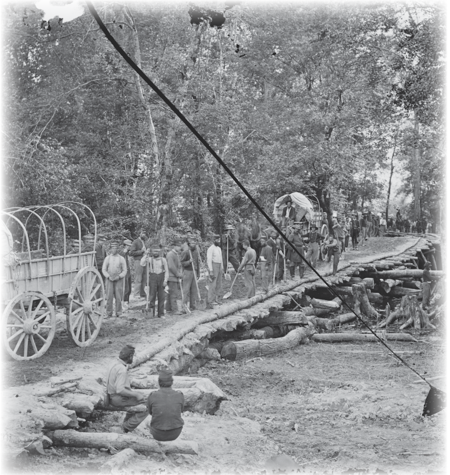
Chickahominy River, Virginia. Grapevine Bridge built May 27-28, 1862, by the 5th New Hampshire Infantry
