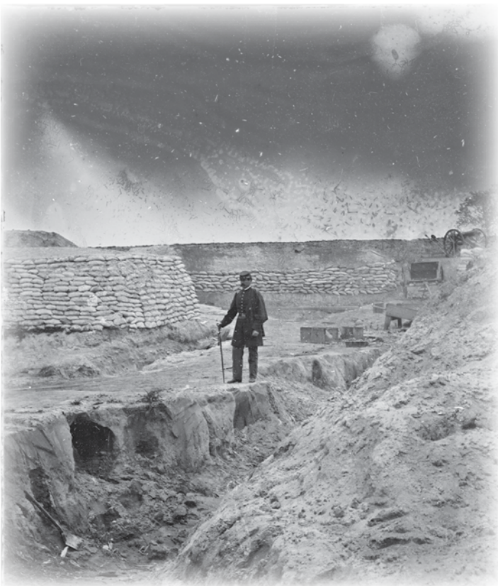
Confederate fortifications, Yorktown, Virginia, 1862. Confederate Gen. John Magruder improved upon the entrenchments erected by Cornwallis in 1781.
