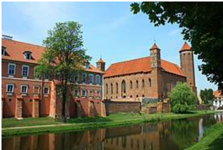
The Warmian Castle Today—the Towers Are 14 Storeys High
