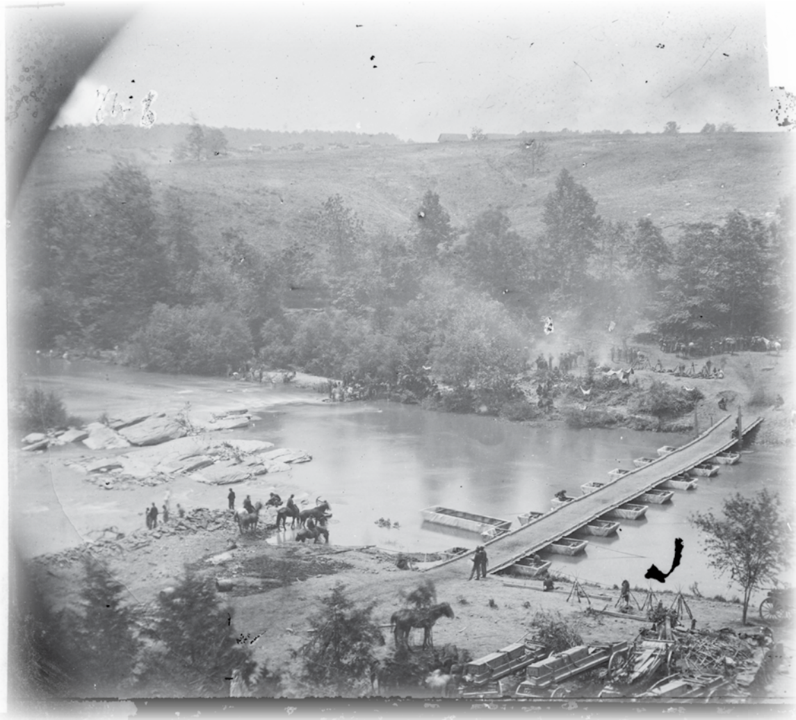
Jericho Mills, Virginia, canvas pontoon bridge, North Anna River. The Union's V Corps crossed here on May 23, 1864.
